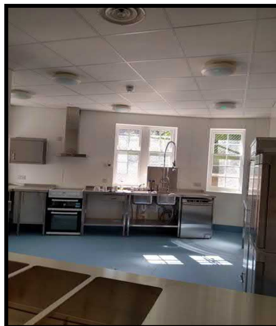
The new downstairs kitchen looking from the serving hatch
